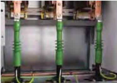
AIS20 with mechanical cable lug
